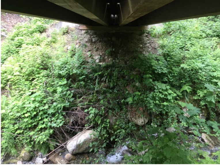
Right Bank Abutment when facing downstream
