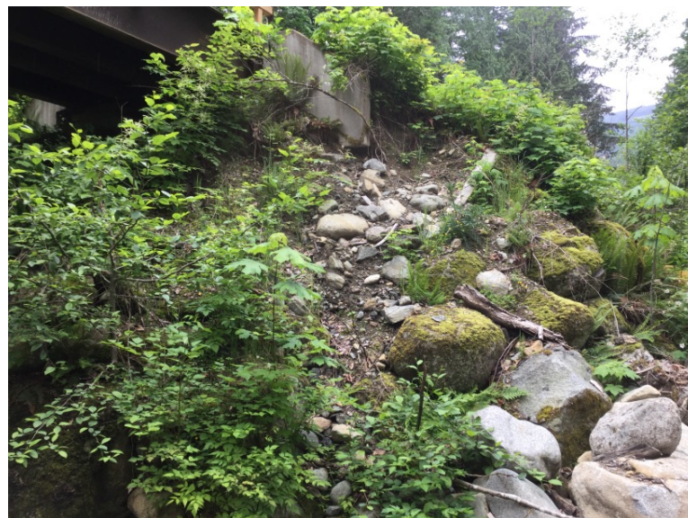
Downstream left bank fill
