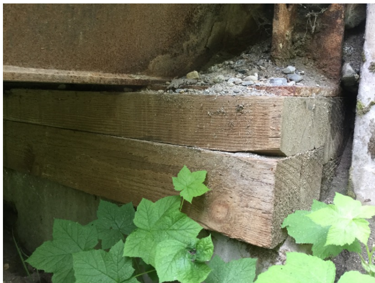
Timber sills stacked at right bank
