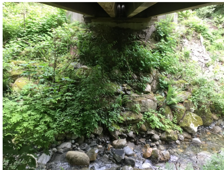
Left Bank Abutment when facing downstream
