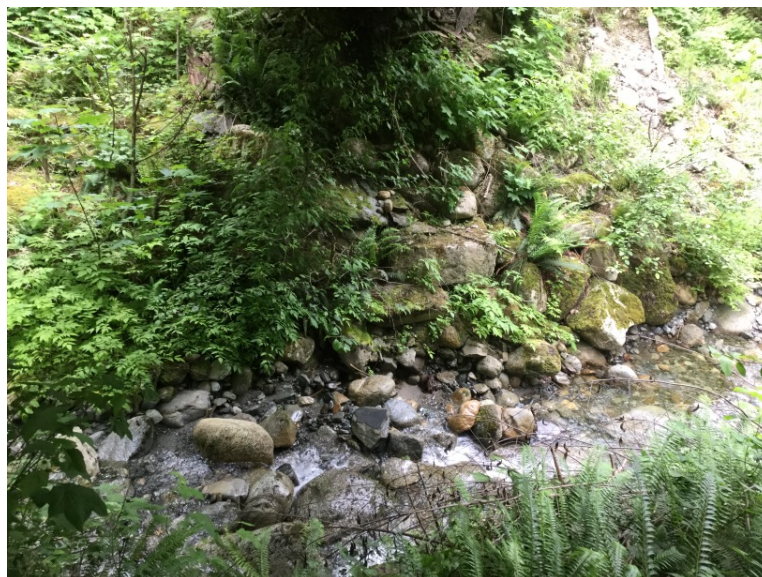
Left bank riprap
